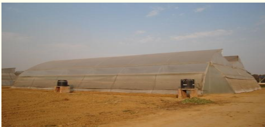
Protected structure: Naturally Ventilated Polyhouse
